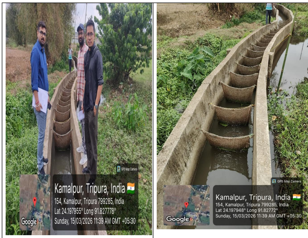
Plate 2: Secondary Treatment-Biological
